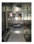
Installed in MV supply substations, the IVision TSTC is the communication interface between the production facility and the SCADA through the DEIE.
