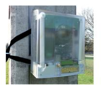
Directional and Amperometric Fault Passage Indicators or Fault Current Indicators for medium voltage overhead and underground networks.
