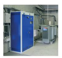
Device for independent electric energy producers preventing the attenuation of pricing control signals sent by the distributor at HVB/HVA source stations.
