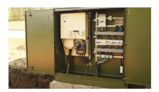
Empty or equipped cabinets with LV public distribution system connection equipment and public lighting control equipment.
