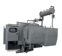
Transformer with automatic voltage regulation system for industrial installations.
